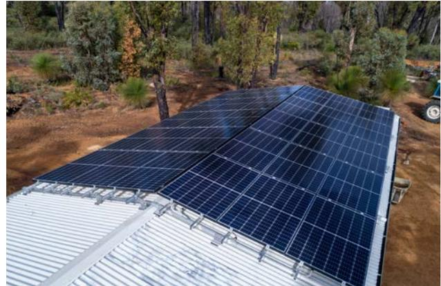
9kW PV array east-west configuration designed to maximise solar yields
