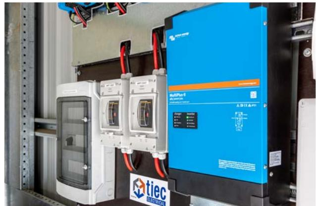
5kVA Victron MultiPlus-II Inverter/Charger, plus PV isolation board and breakers.
