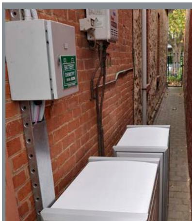
At Mr Altree-Williams' renovated 100-year-old College Park bungalow, ZCell installer Off-Grid Energy installed an energy storage system with two ZCell zinc-bromine flow batteries, with a total energy storage capacity of 20 kilowatt-hours (kWh), supported by two Victron MultiGrid 48/3000/35-50 battery inverter-chargers. The batteries receive energy from 27 Tindo 270-watt photovoltaic solar panels, connected to two Victron BlueSolar MPPT 150/70 solar charge controllers.
