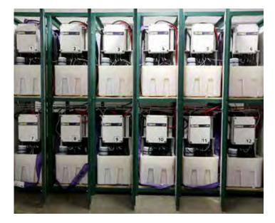
Bosco Printed Circuits Director Mr Philip Verheul said the company installed the Redflow batteries to avoid loss of production. "In our process, we have electroplating lines in which we plate copper in holes, so if there's a power failure during the process. everything in the line is basically scrapped," he said.
